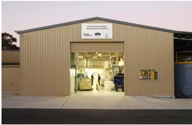
Main DPP Shed
