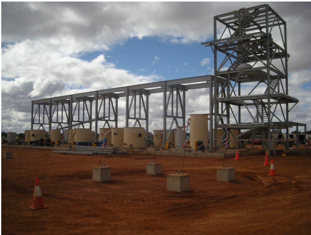
Steelworks erected above the flotation building at the Concentration Plant, Western Australia
